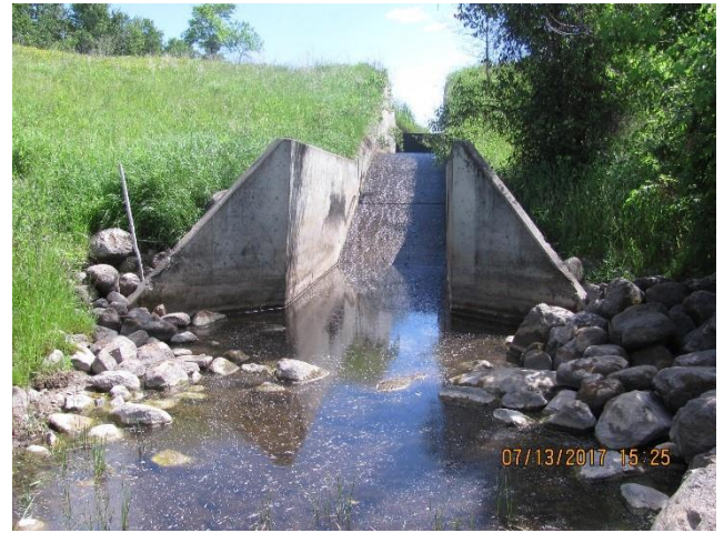
North Branch Drop Structure – JD 31
