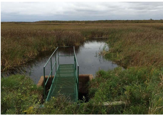
Outlet Structure – Horseshoe Lake
