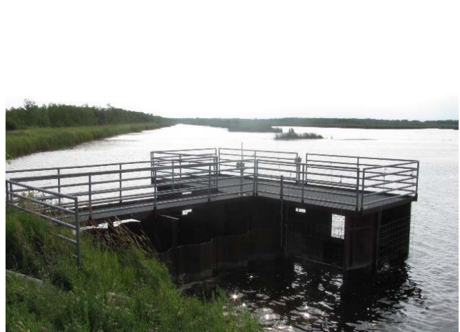
Main Outlet Structure at Nereson Impoundment
