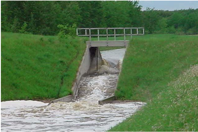
North Branch drop structure – SD 84
