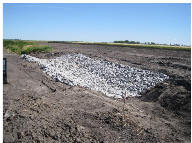
Grade Stabilization – Springbrook #10
