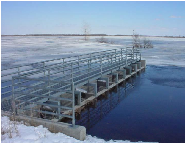
Outlet Structure at Ross #7 Impoundment
