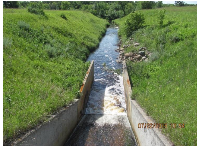
North Branch Drop Structure
